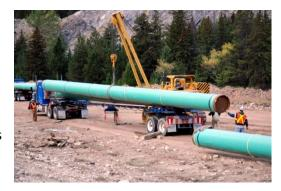
**Nipisi Pipeline:** 100 km of NPS 24, 90 km of NPS 20, and 145 km of NPS 8 diluent and warm temperature blend oil pipelines located in northwest Alberta. The engineering scope of work included routing studies, detailed design, construction contract documentation, and engineering support during construction.
