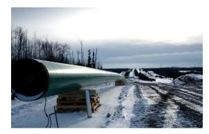
**Corridor Pipeline Expansion**: 463 km of NPS 42 pipeline for complete EPCM services, including detailed engineering design, procurement, construction contract documentation, construction inspection, construction management, and engineering support during construction. The project included winter and summer construction through a range of muskeg swamp, rolling bushland, and developed farmland.
